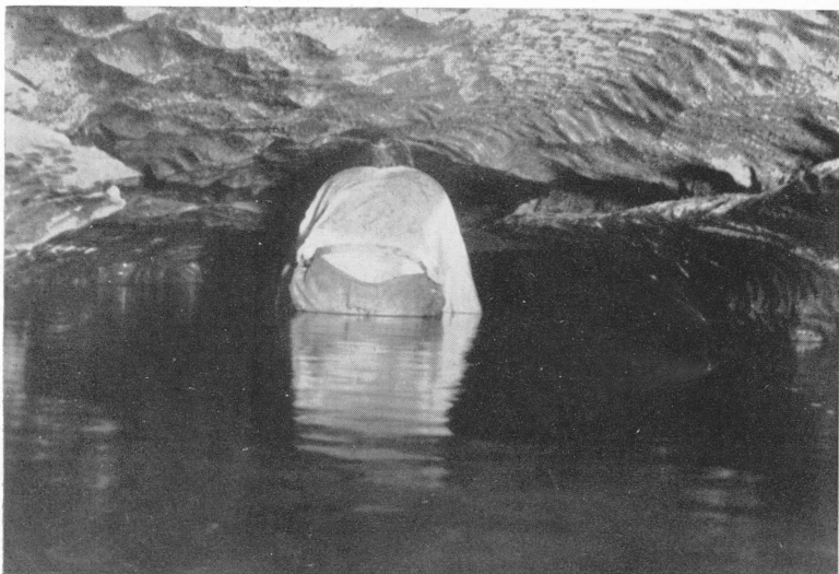
A. —The Canal. Photograph taken near cross-section 3, looking upstream.
