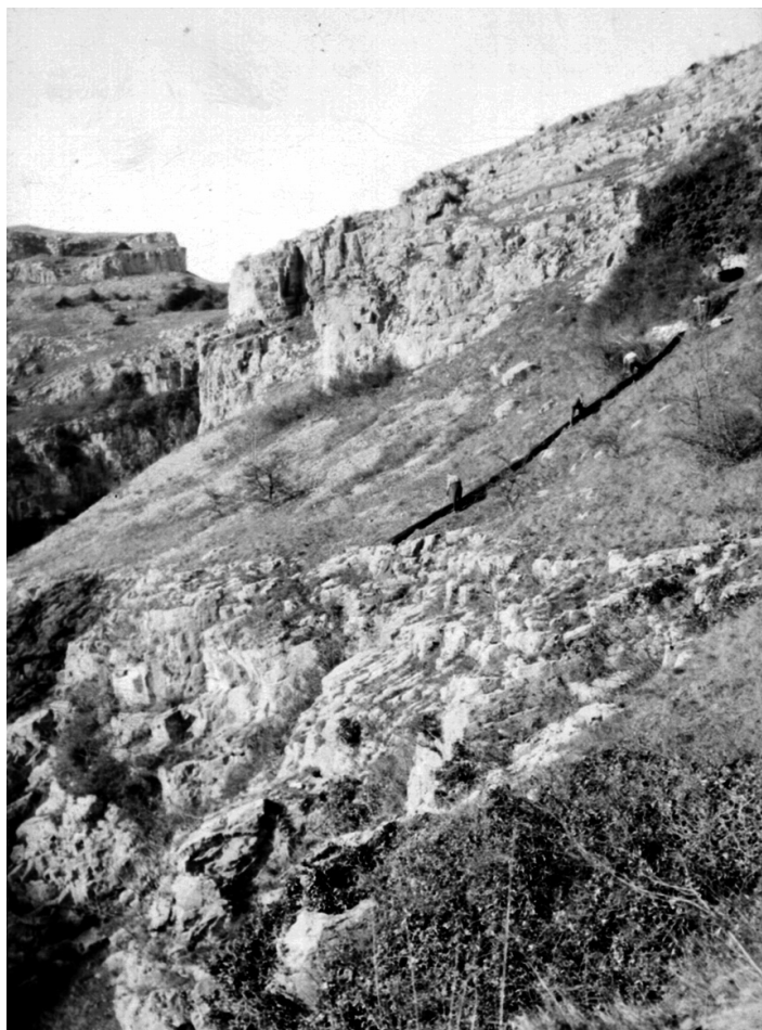
Figure 6. Sun Hole, 1927. The chute for disposing of spoil.
