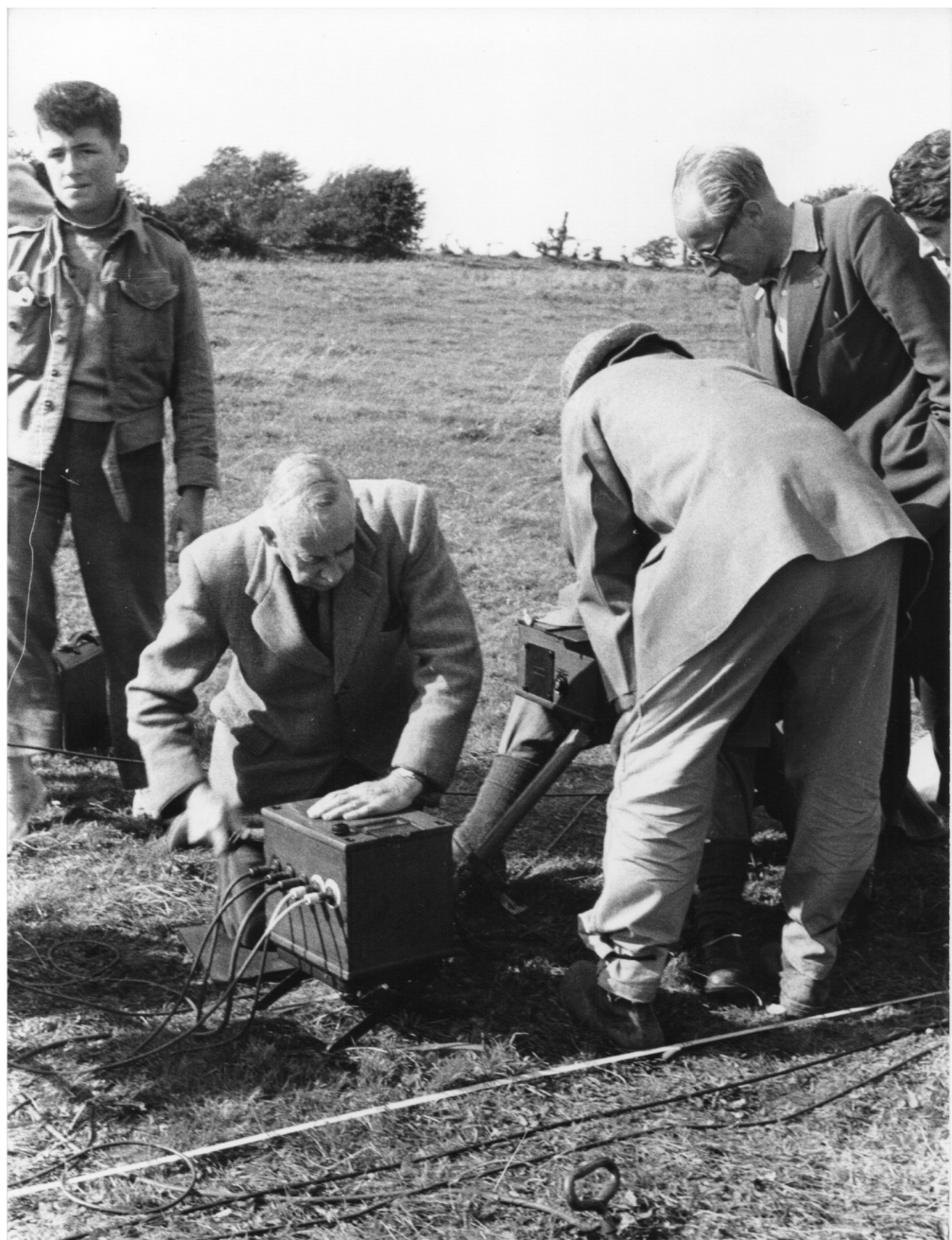
Figure 1. The Megger earth tester in use over Lamb Lair, 1956. The kneeling figure (L.S. Palmer) is hand cranking the generator and the two other figures are looking down on the galvanometer.
