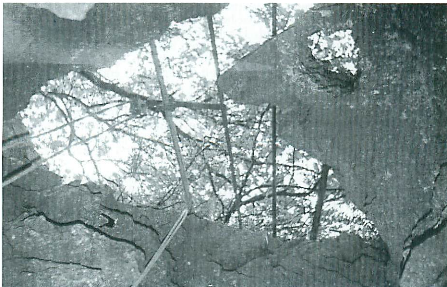
FIG. 4—VIEW SKYWARDS AFTER REMOVAL OF INFILL. NORTH IS TO THE RIGHT-HAND SIDE, SOUTH TO THE LEFT-HAND SIDE Phot.: A. G. Clarke
