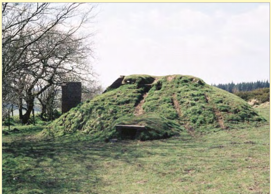
The west control room showing the blast wall and also one of the outlets for control cables.
